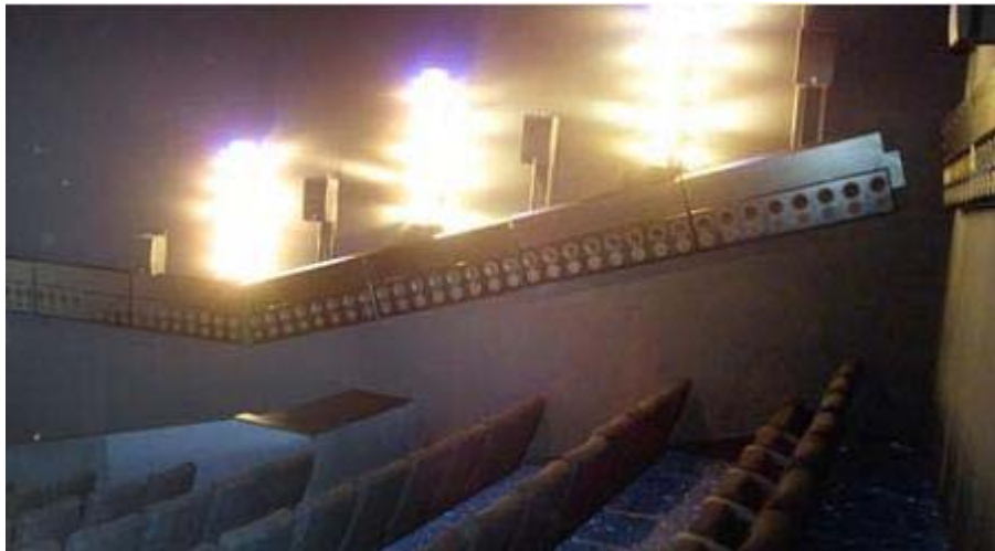
Fig. 4.16 A WFS cinema system in Ilmenau
