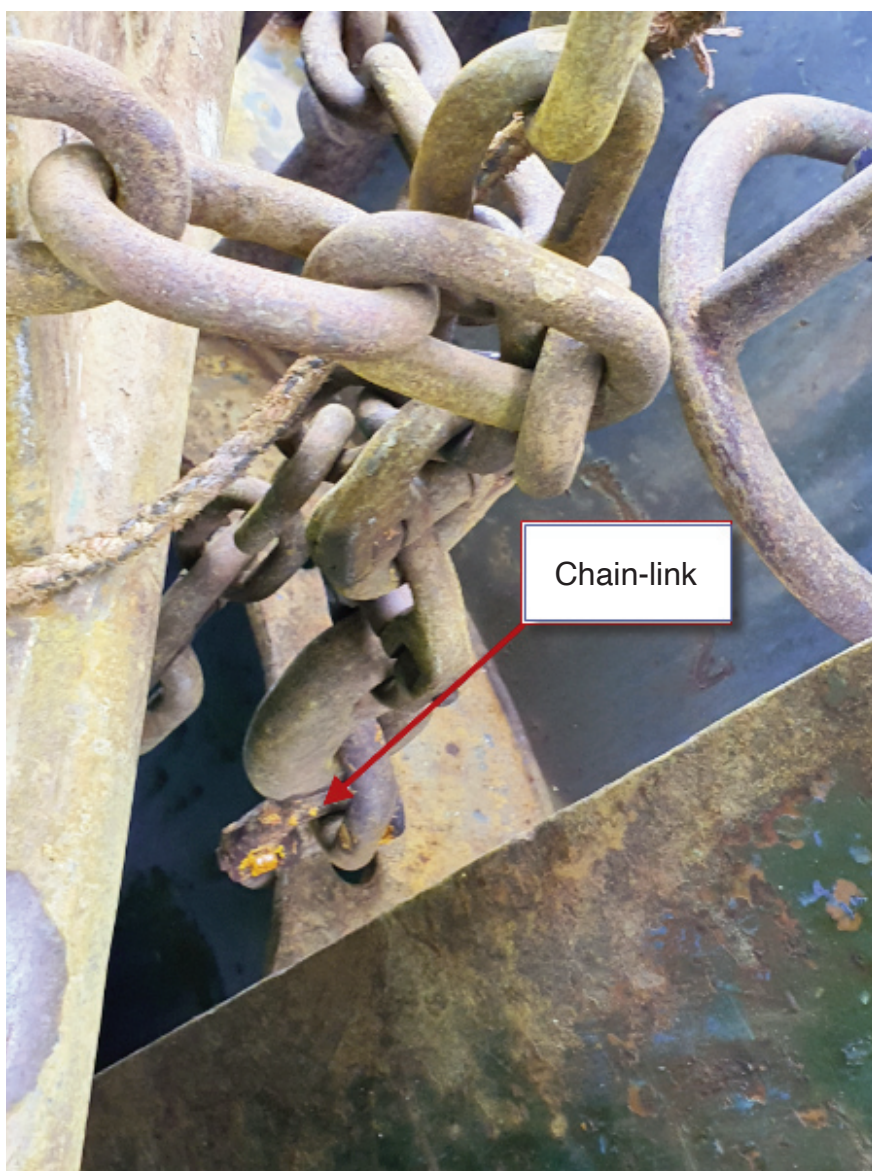
Appendix 7.14 Photograph No. 6 - Chain-link
