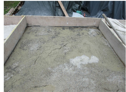
(d) The assemblage slakes for three or four days covered with fabric.
