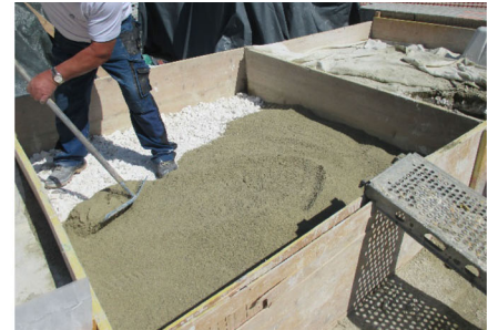
(b) The layer of quicklime is then covered with a second layer of sand.
