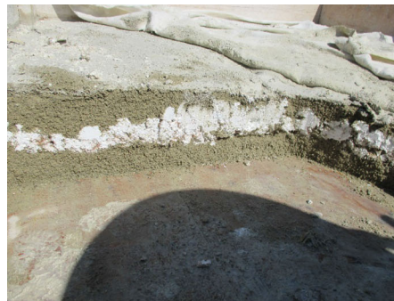
(e) The mortar is prepared with the cooled, slaked lime. When preparing the mortar, the masons shovel across the pile to pick up all the layers.
