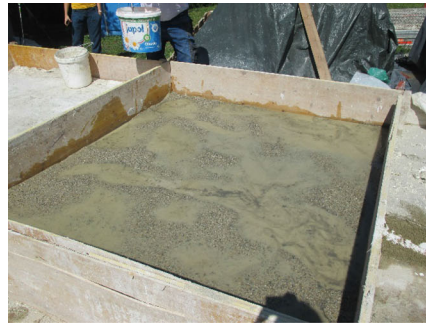
(c) Water is sprinkled to initiate slaking.
