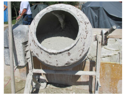
(f) Finally, standard mixing is carried out in a paddle or drum mixer, and water is added to achieve the desired consistency.
