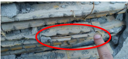
Figure 12: Splitting of tension bamboo.
