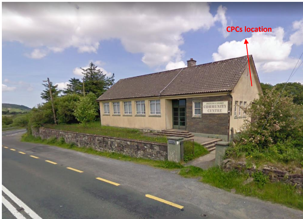
Figure 3. 2 Demo-site Mayo, Ireland at Brackloon Drummin Community Centre
