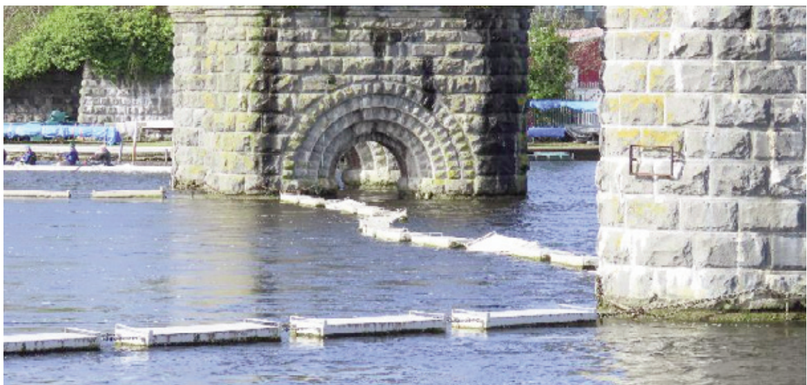
Figure 15: The safety boom protection, 100 m upstream from the Salmon Weir.
