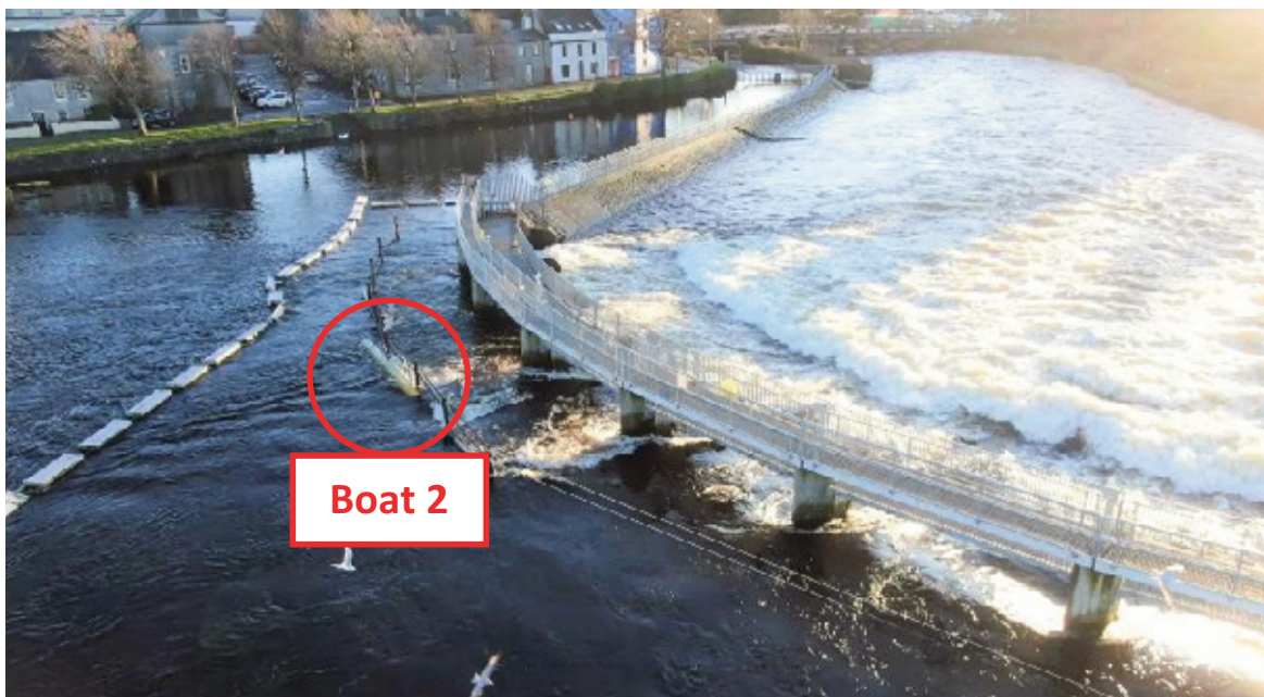
Figure 39: Boat 2 on the chains immediately above the weir. Source: Galway Aerial Cinematography
