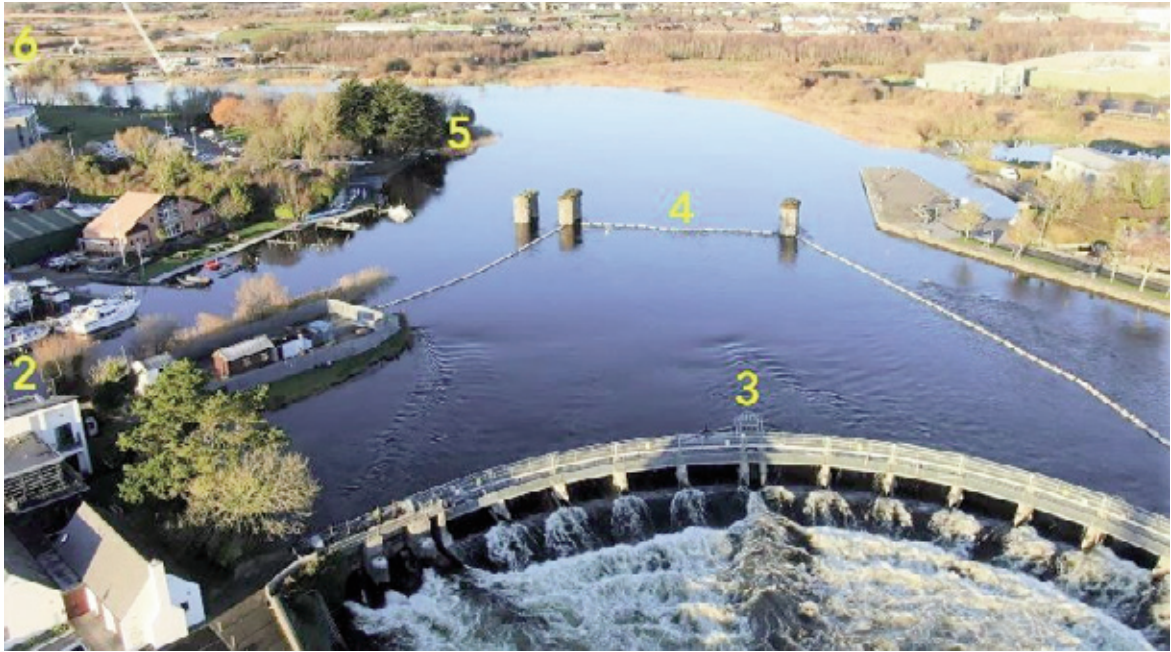
Figure 27: Aerial overview of part of section of river where this casualty event occurred. Viewed looking north, showing: 2. The Eglinton Canal; 3. The Salmon Weir; 4. The weir's safety booms; 5. The Jes corner; 6. Quincentennial Bridge. Note: University of Galway Boat Club's boathouse (1) is out of view, to the south of Eglinton Canal (2). Source: Galway Aerial Cinematography.
