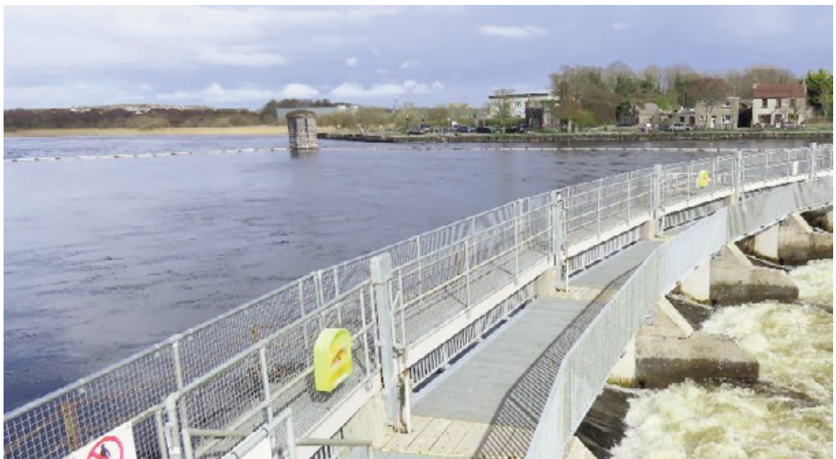
Figure 13: The enclosed water, extending 100 m upstream from the weir.
