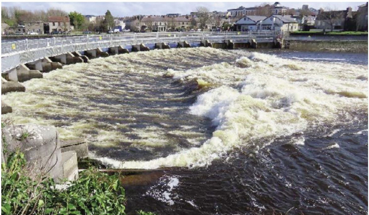
Figure 6: The Salmon Weir during winter flow conditions (in March 2023), when all 16 sluice gates are open.
