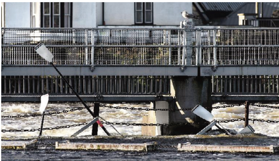
Figure 40: Oars from this casualty event on the chains immediately above the weir. Source: Joe Shaughnessy/Connacht Tribune
