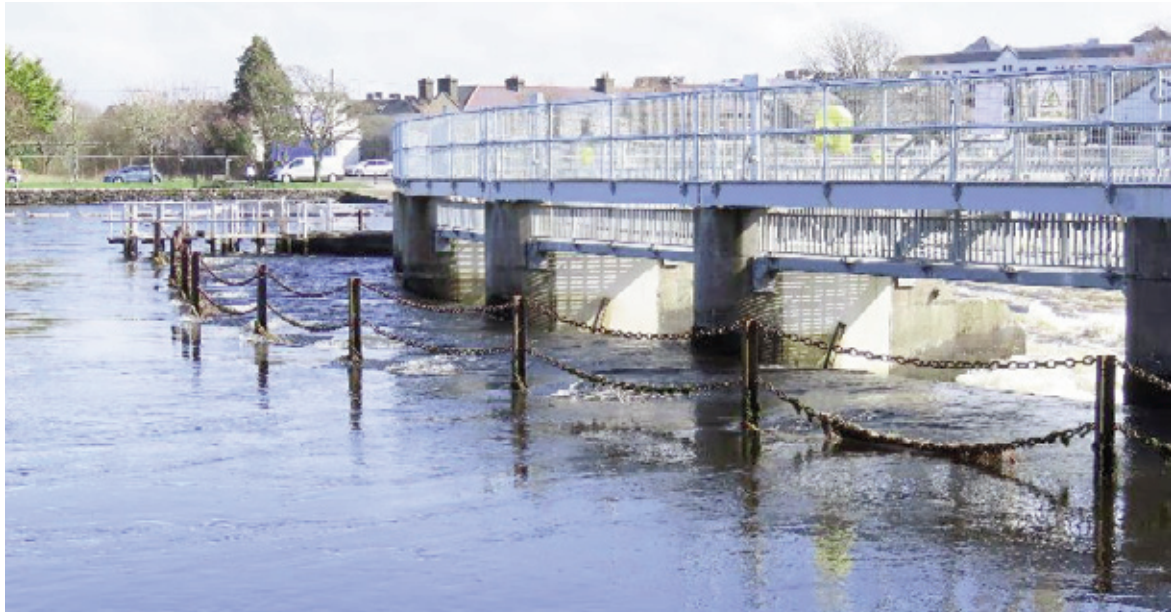
Figure 12: The chain protection, immediately above the Salmon Weir. Viewed from upstream.
