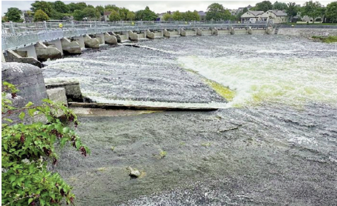
Figure 7: The Salmon Weir during summer flow conditions (in August 2023), when only two of the 16 sluice gates are open.
