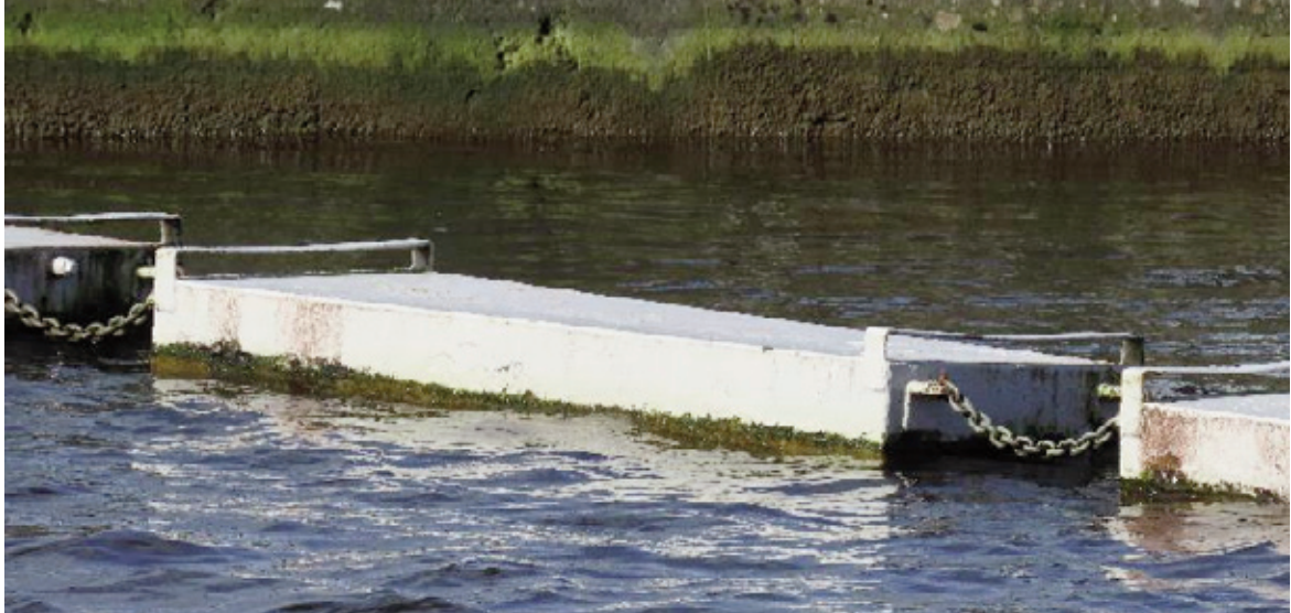
Figure 14: Example of the safety boom in place above the weir.
