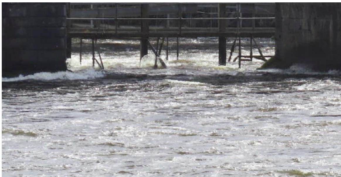
Figure 9: The river-wide obstacle at the Salmon Bridge, viewed from upstream.
