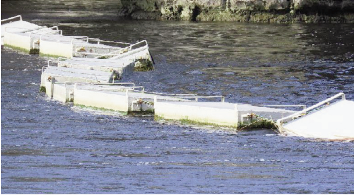
Figure 16: The safety boom protection, 100 m upstream from the Salmon Weir.
