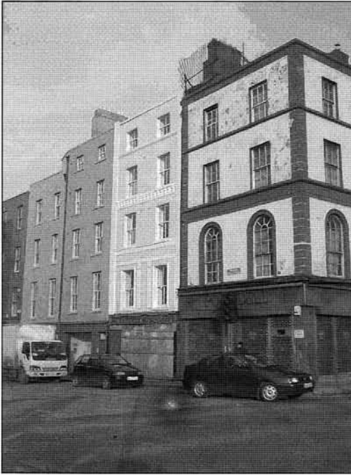
Figure 3. Numbers 2 and 3 Capel Street, Dublin, after refurbishment (Negussie, 2002)
