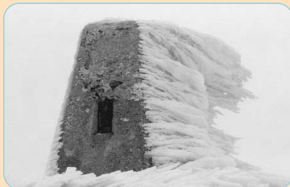
ii) Rime, or ice accretion, growing on an Ordnance Survey pillar on Slieve Donard
