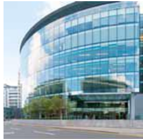
Central Park Grade A Office, Landlord fit-out
