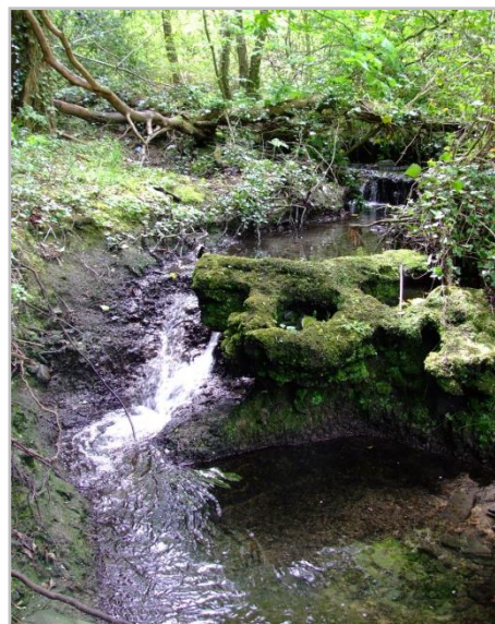
Photo 29: Eroded dam a short distance downstream of Photo 28 (May 2013).
