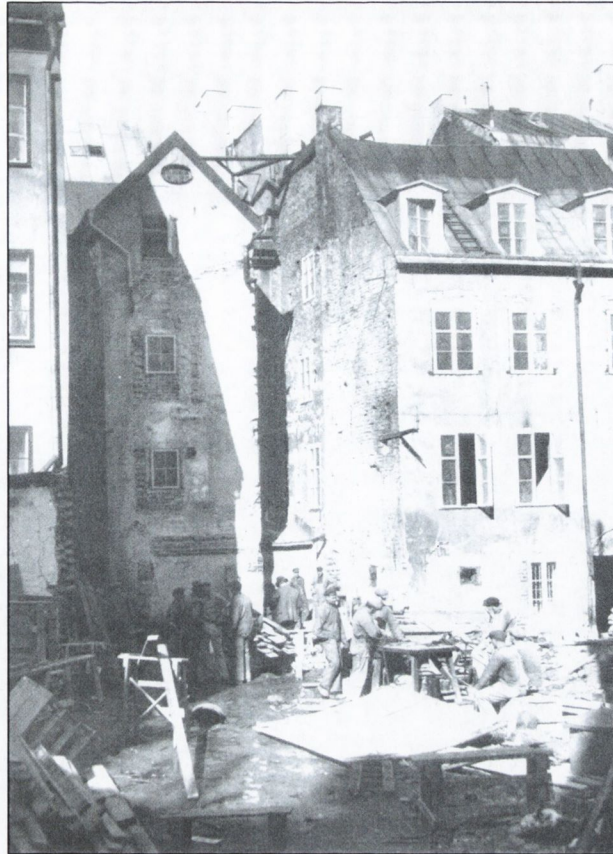
Figure 8.23: Refurbishment of the Cepheus Quarter (Svenska Dagbladet, 1973, Stockholm City Museum).
