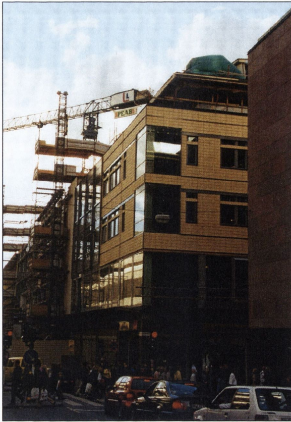
Figure 8.32: The same building as in figure 8.31 (Negussie, 2001).
