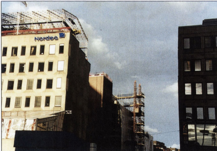
Figure 8.33: Further evidence of a new trend for floors to be built on top of existing modern buildings in Stockholm City (Negussie, 2001).
