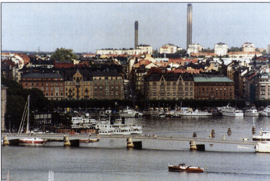
Figure 8.19: The Skeppsholmen Bridge (Negussie, 2001).
