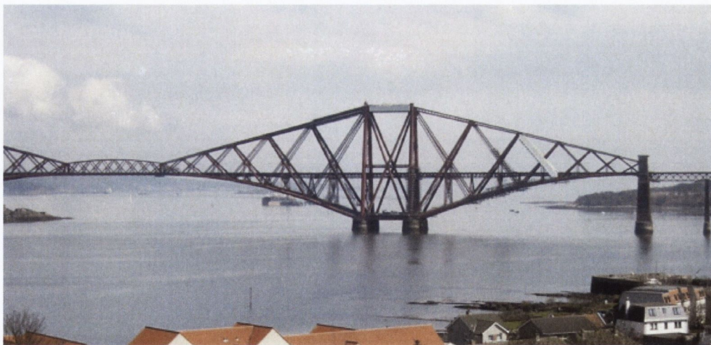
Figure 4.5 – a truss bridge
