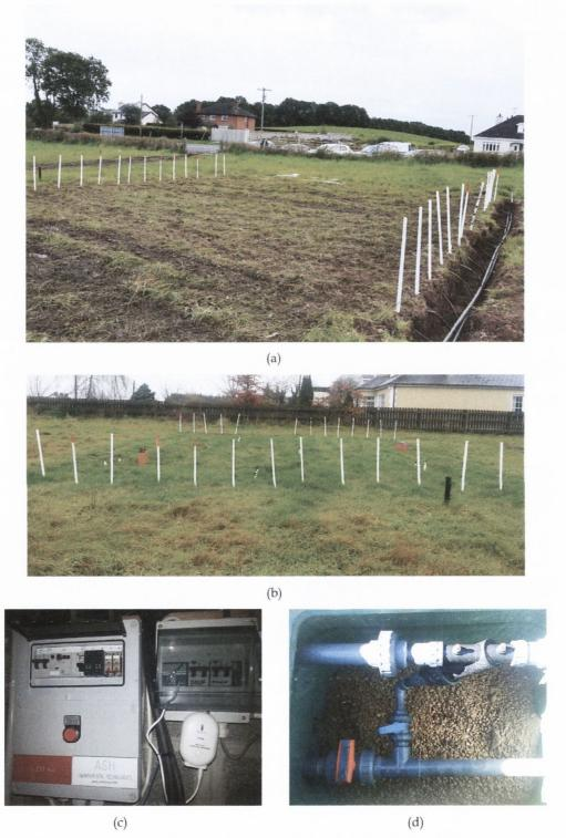
**Figure 4.22** (a) Installed driplines and supply/return manifolds, (b) completed DD system 4 weeks after installation, (c) DD control panel with installed Elink meter and (d) filter for DD system
