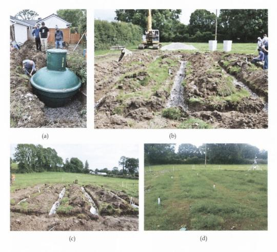
Figure 4.20 (a) Installation of ASP unit at Site A (August 2012), (b) construction of LPP gravel trench, (c) geotextile in LPP trench and (d) complete LPP trenches 4 weeks after installation (September 2012)
