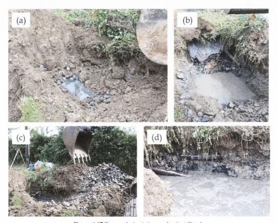
Figure 6.17 Removal of existing soak-pit at Site A
