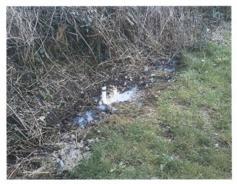
Figure 6.4 Effluent ponding at surface of drainage ditch
