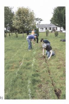
Figure 4.21 (a) Installation of Clereflo filter unit at Site B and (b) installation of driplines by hand
