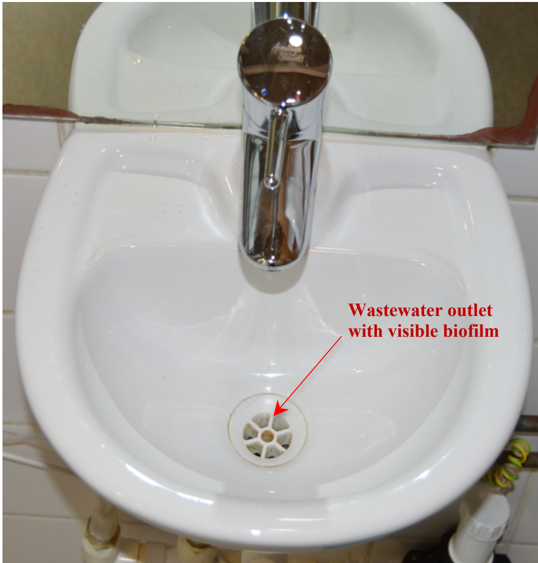
Figure 1.5 Photograph showing a washbasin drain outlet contaminated with visible biofilm . It can be clearly seen that the biofilm from the U-bend reaches the sink drain outlet.
