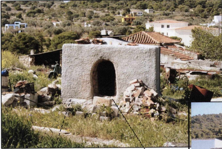
Front of Kiln- Opening for Loading and unloading Kiln
