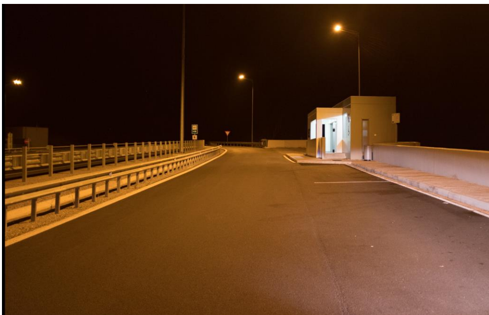
Figure 12 A motorway pull-in area in Greece illuminated by 1750K Amber LED. This is a NATURA 2000 area. The visibility levels are acceptable and the colour rendering is more than acceptable.
