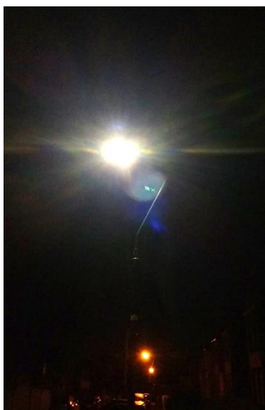
Figure 10 (left) This image shows an LED replacement for a SOX unit on an angled bracket of larger angle than can be accommodated by the luminaire tilt setting; (right) The image at right shows the brightness of a single LED lamp replacement amongst high pressure sodium lighting on the outskirts of a town. The striking brightness and glare of the LED lamp – both direct and via the wet road – is apparent. Note that the lighting levels in this instance were not well matched.
