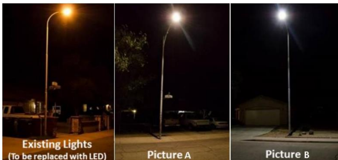
Existing 2200 Kelvin HPS
