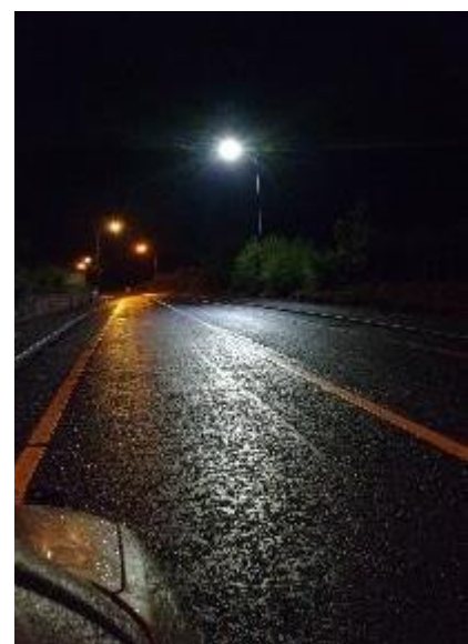
Figure 10 (left) This image shows an LED replacement for a SOX unit on an angled bracket of larger angle than can be accommodated by the luminaire tilt setting; (right) The image at right shows the brightness of a single LED lamp replacement amongst high pressure sodium lighting on the outskirts of a town. The striking brightness and glare of the LED lamp – both direct and via the wet road – is apparent. Note that the lighting levels in this instance were not well matched.
