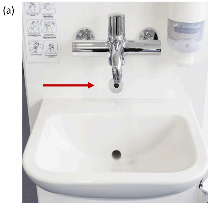
Figure 1.2 Photographs showing examples of a DP and a HP washbasin in DDUH. Panel (a) shows an example of a HP washbasin located in Clinic 2. The washbasin lacks an overflow outlet, has an offset drain outlet and the tap is operated by a motion sensor indicated by the red arrow. The tap is equipped with a thermostatic mixing valve and is configured to provide output water at an average temperature of 38°C to prevent scalding. Panel (b) shows an example of a DP washbasin located in West Clinic. The tap water flow directly impacts the drain outlet and the washbasin has an overflow outlet. The washbasin is equipped with a manual mixer tap. Tork Extra Mild Liquid Soap (SCA Hygiene Products Ltd., Bedfordshire, UK) (non-medicated) is the only soap used for handwashing in DDUH.
