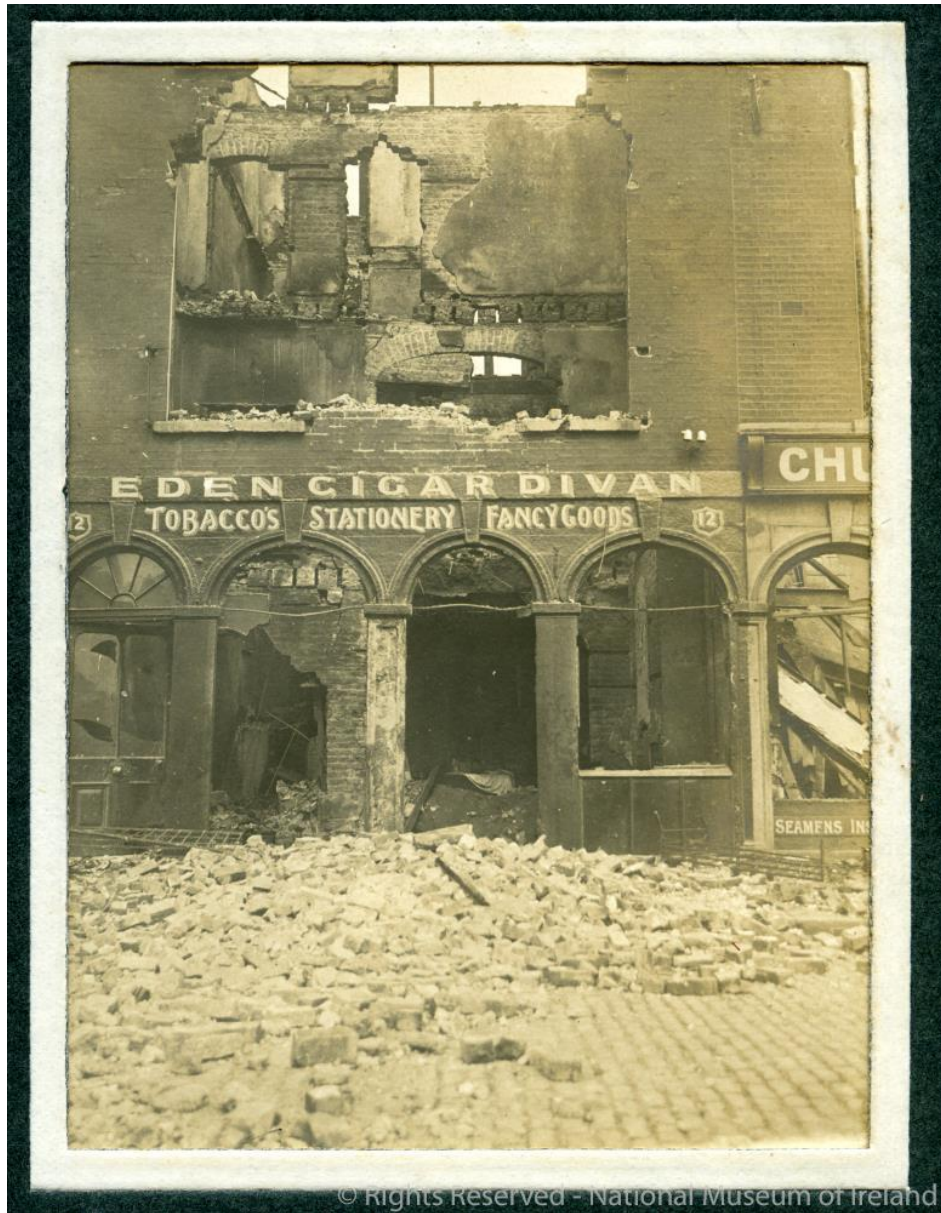
Figure 5: The ruins of 12 Eden Quay in 1916, showing Joseph Corringham's tobacconist shop at street level, and the broken skeleton of Emily Dalby's lodging-house above. To the right is the Seamen's Institute, where Emily's father worked. 176
