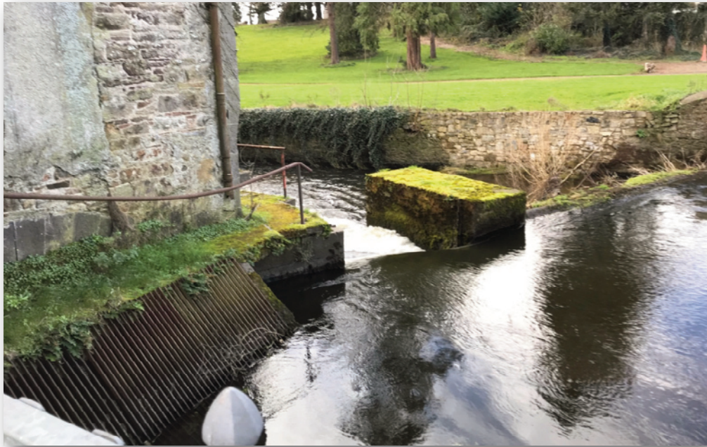
Photograph No. 7: Weir where the capsizing occurred.
