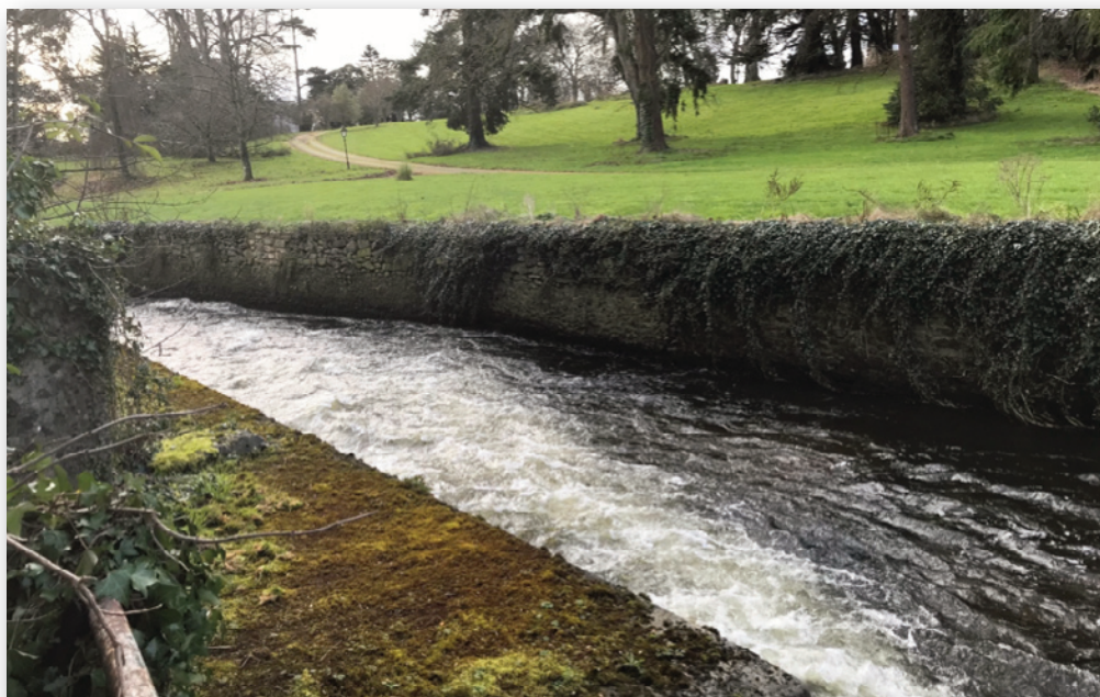
Photograph No. 9: Rapid flowing water downstream from weir.
