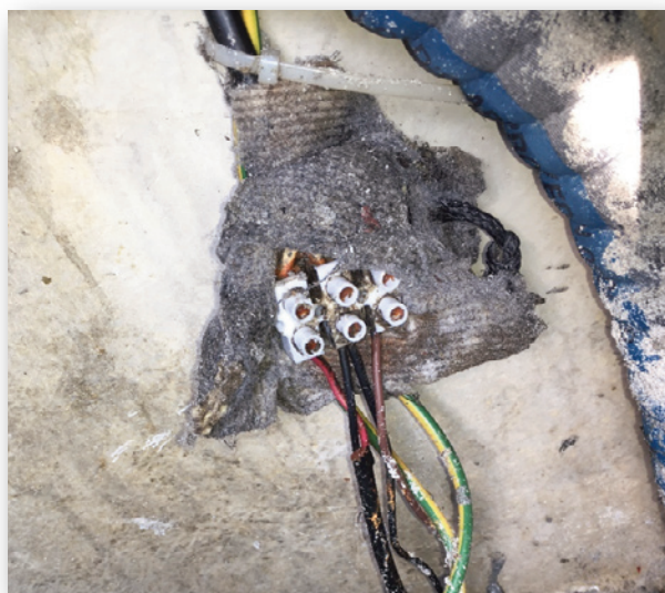
Photograph No.8 - Electrical connections to the bilge pumps in starboard engine compartment.
