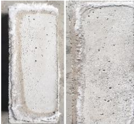
Figure 8. Efflorescence in \text{Na}_2\text{SiO}_3 activated GGBS cured in ambient conditions probably due to a high \text{Na}_2\text{O} content in the mix.
