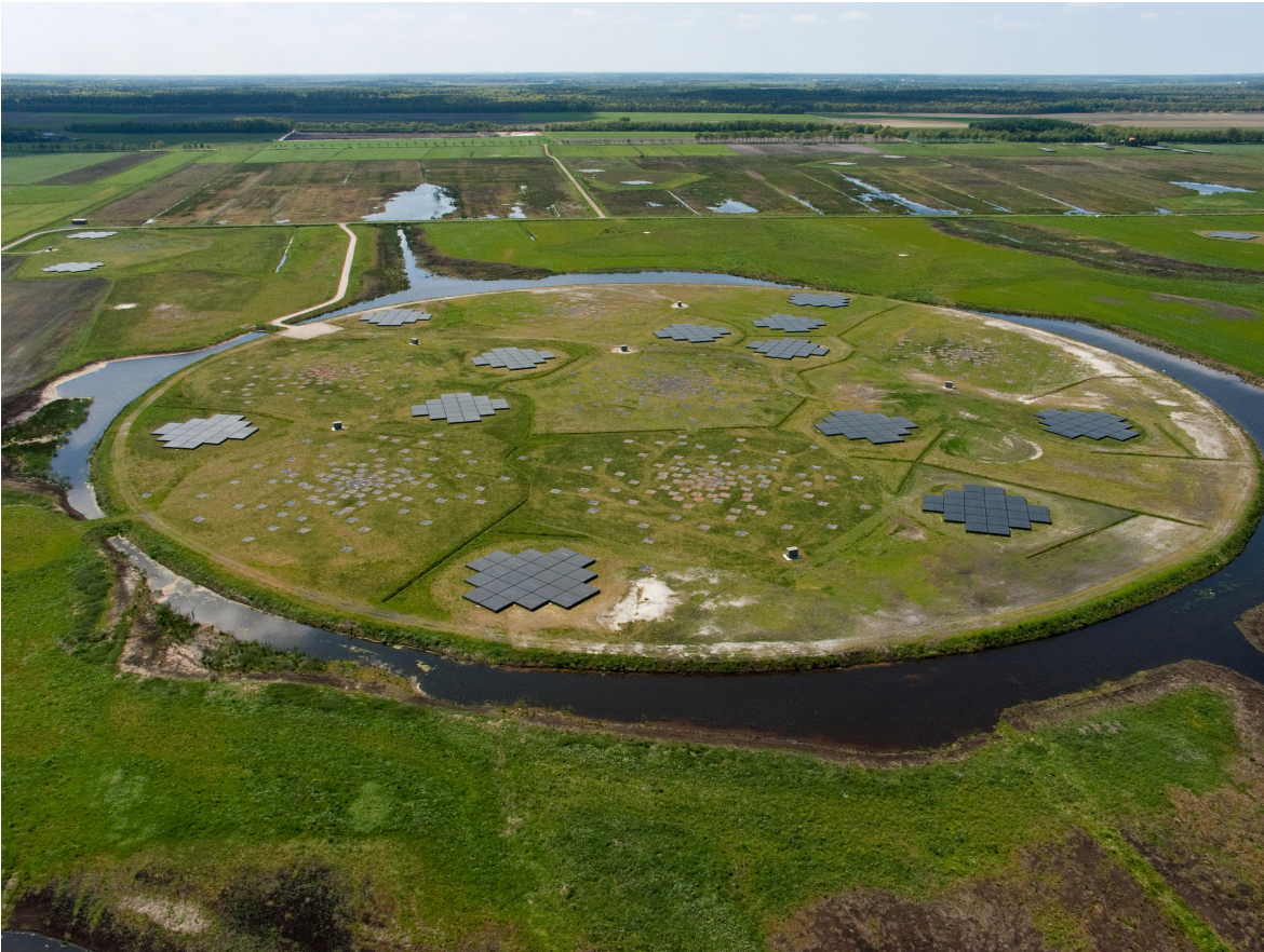
Figure 3.1: A dense collection of LOFAR core stations known as the “superterp”. The large black tiles are the HBAs while the smaller grey squares mark the locations of the LBAs. A moat is dug around the superterp to keep the antennas above the ground water. Image credit ASTRON/LOFAR.
