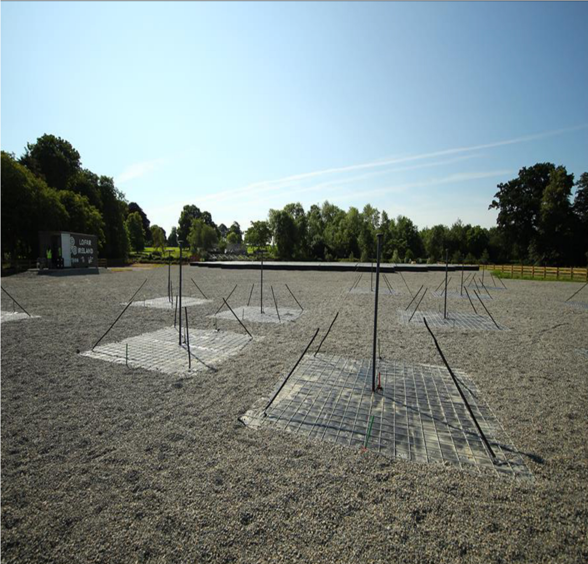
Figure 3.2: Low Band Antennas on a rare sunny day at I-LOFAR. These dipole antennas observe between 10 and 90 MHz. The dipoles are connected to a preamplifier on top of a PVC pipe via coaxial cables which run underground to the station container in the background.
