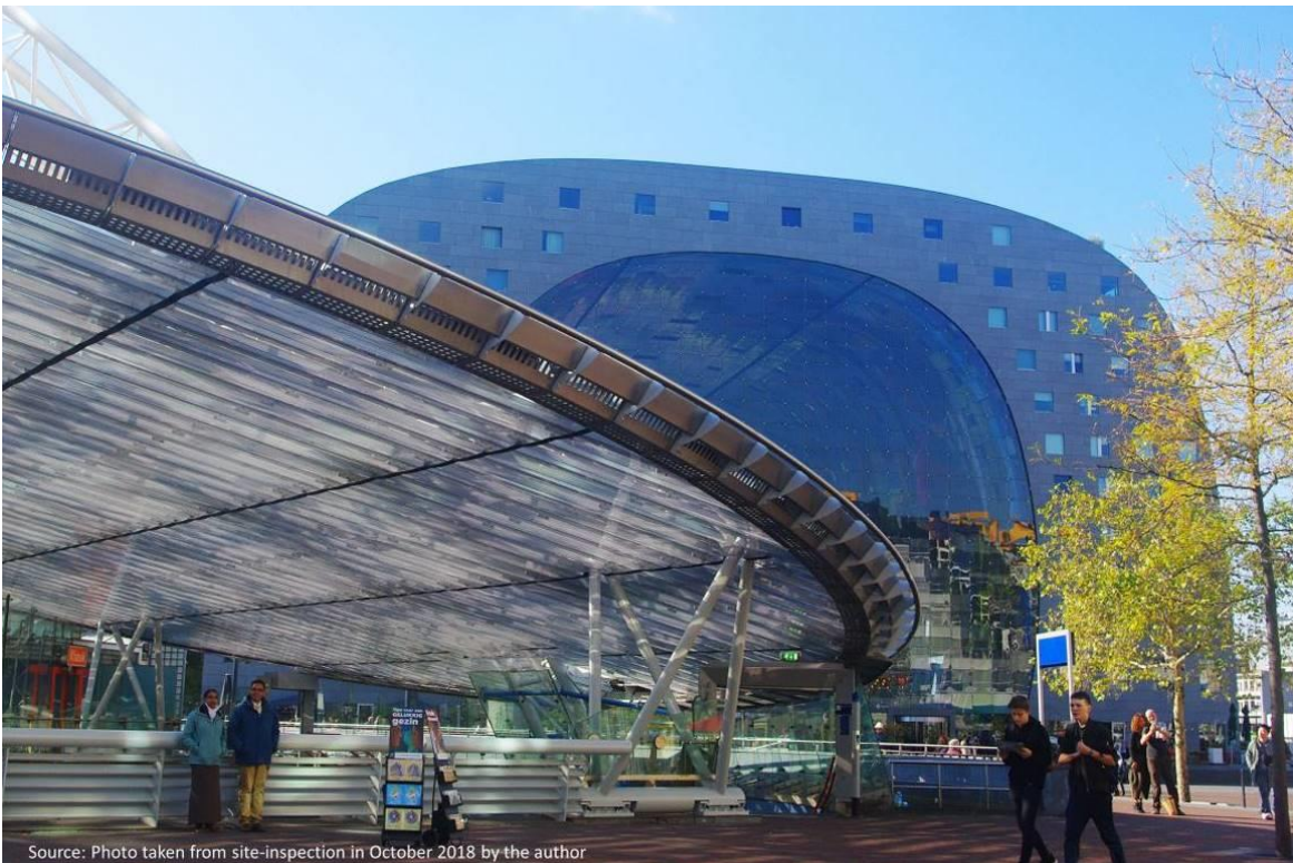
Figure 6-7 Rotterdam inner city near the old harbor; the markthal is a new landmark of Rotterdam
