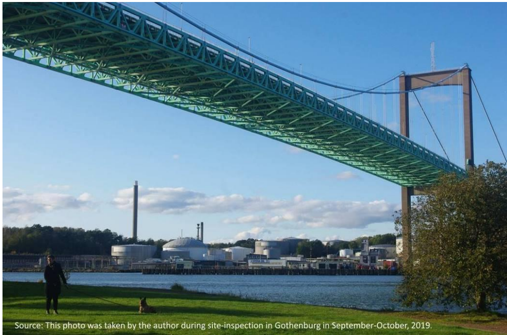
Figure 7-11 Energy port on the North riverside (photo taken from the south, under the Älvsborg Bridge)
