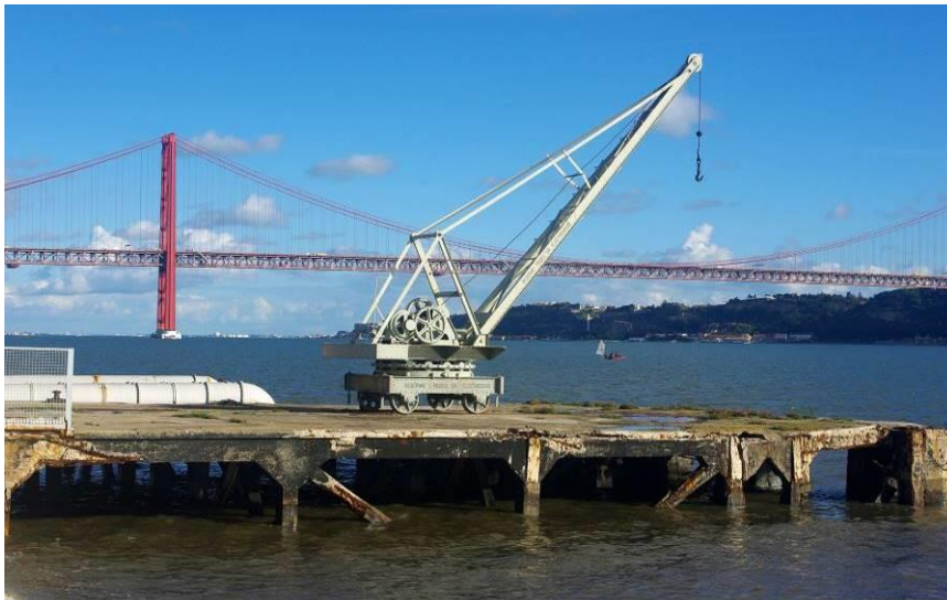
Source: Photo taken by the author during the site inspection in Lisbon in November, 2018
