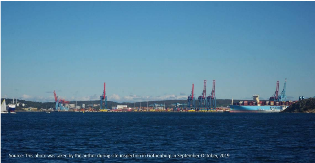
Figure 7-12 Port activities on the way to Gothenburg's archipelago
